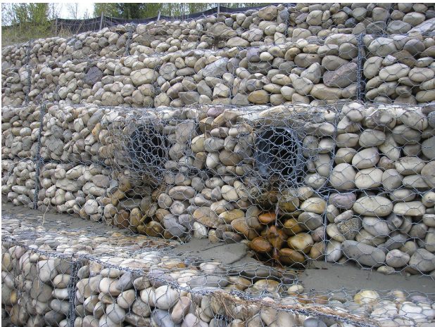
Figure 6. Manhole outlets in gabion outfall structure.
