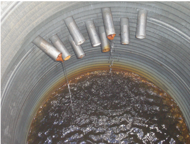
Figure 5. Subhorizontal drain outlets.
