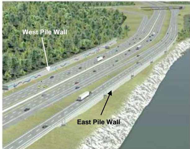
Figure 2. Artistic depiction of upgraded Hwy 63 and East and West Retaining Walls, looking north
