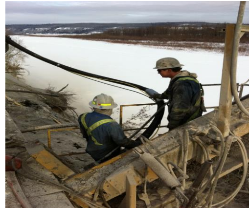
Figure 9. Feeding strands into anchor holes
