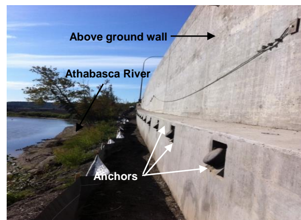
Figure 11. Looking south at the wall from the riverside
