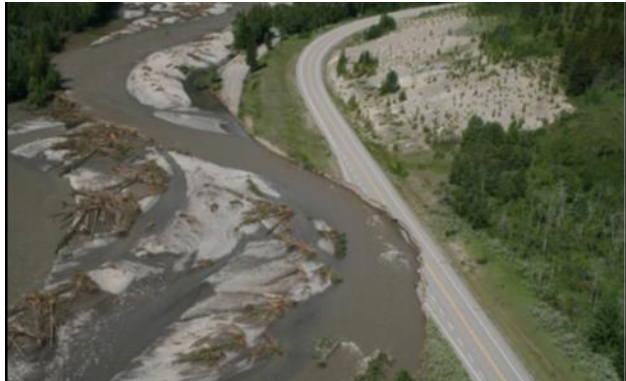
Figure 1. Highway encroachment hazard (AT image).
