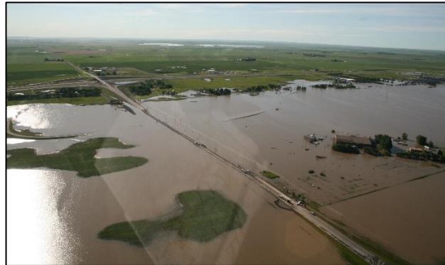
Figure 2. Highway flood inundation hazard (AT image).
