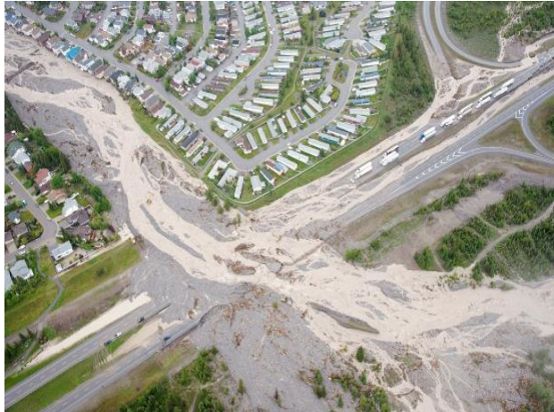
Figure 1. Trans-Canada Highway at the Town of Canmore on June 20, 2013. Photo: Town of Canmore
