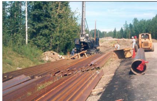
Figure 13: Piling Installation - Lower Level
