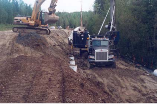
Figure 14: Piling Installation – Upper Level
