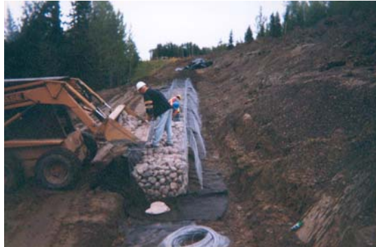
Figure 15: Upper level Gabion Basket Wall
