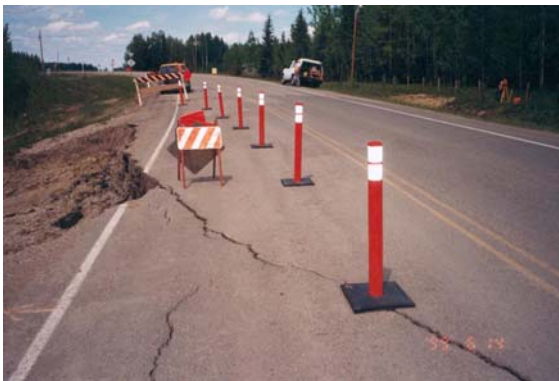
Figure 5: Southbound lane Closure
