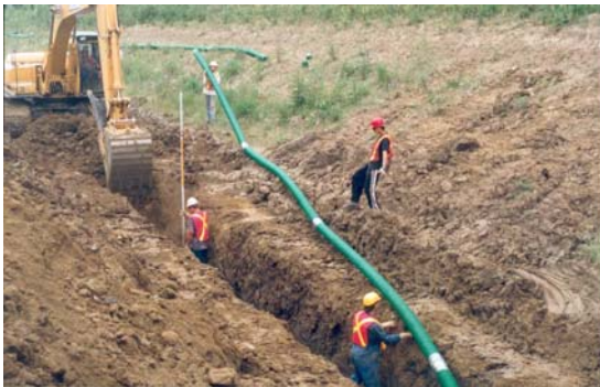
Figure 12: Sub-Drain Installation – Solid Pipe
