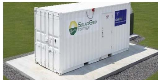
Figure 5 – Modular battery bank – Photo credit – Solar Grid
