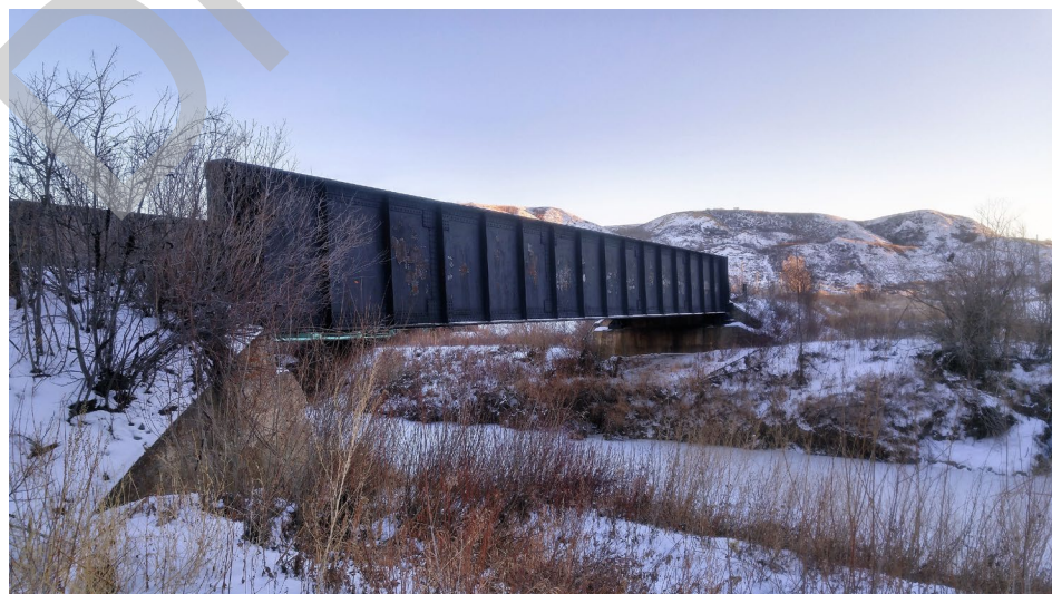
Downstream Side of Bridge
