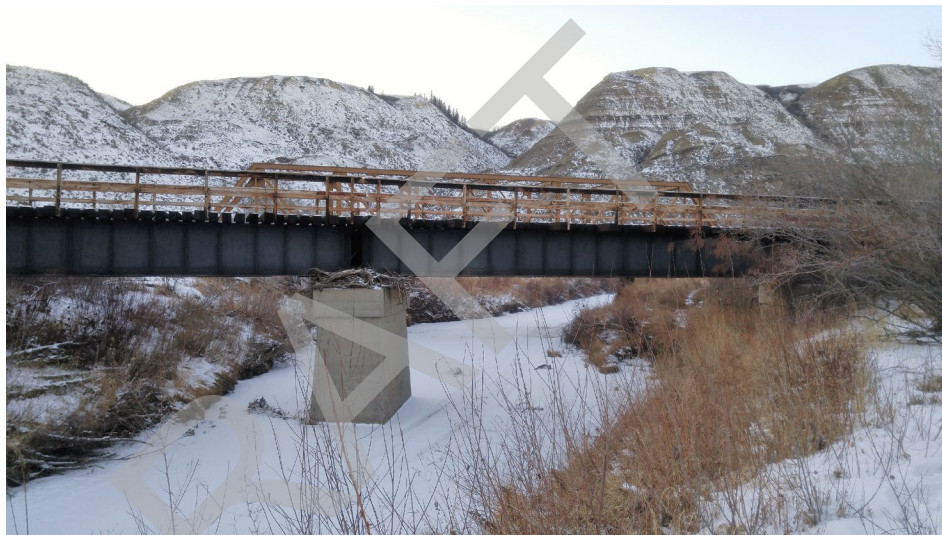
Upstream Side of Bridge
