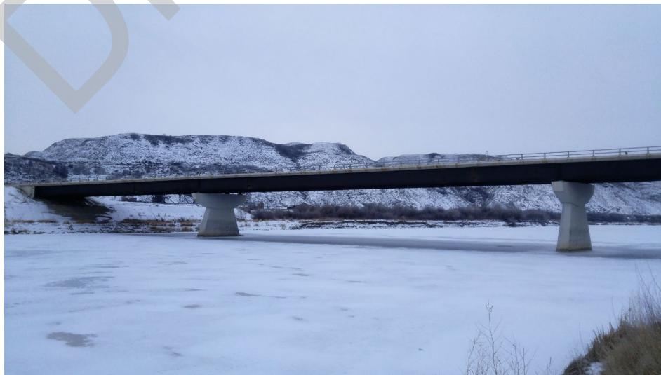
Downstream Side of Bridge
