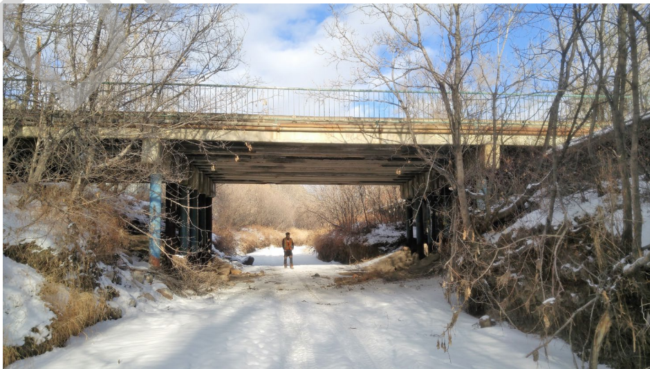
Downstream Side of Bridge
