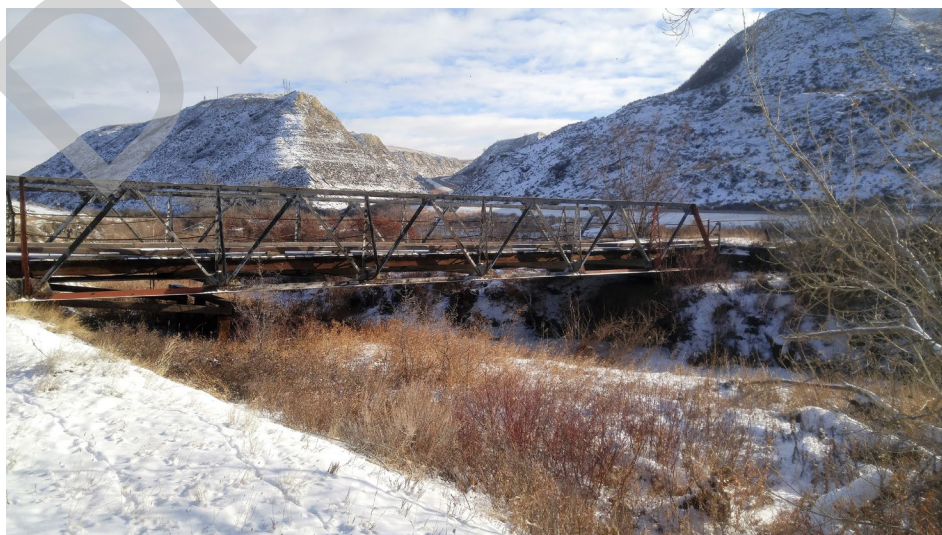
Downstream Side of Bridge
