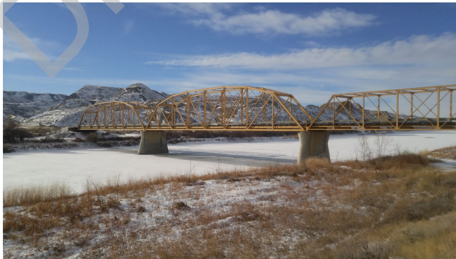
Downstream Side of Bridge
