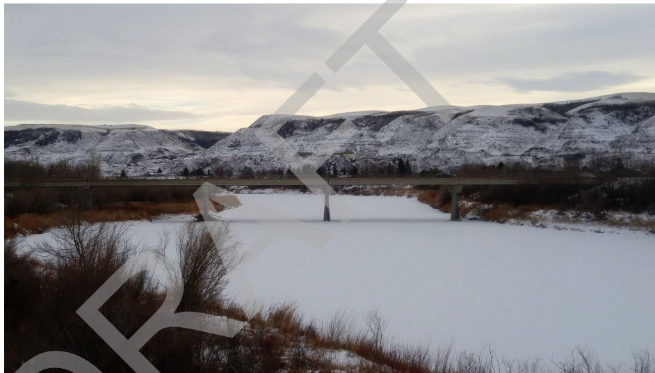
Upstream Side of Bridge
