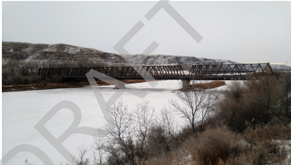
Upstream Side of Bridge
