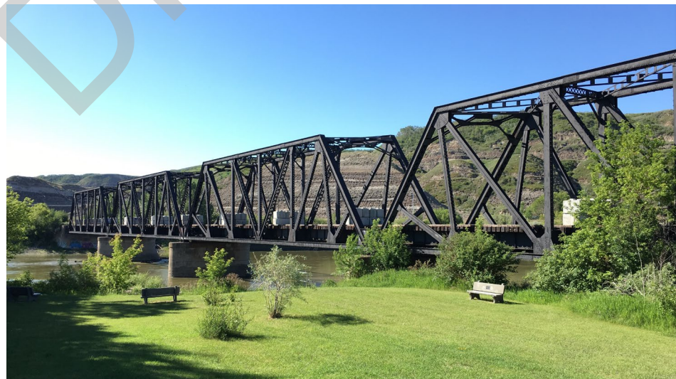
Downstream Side of Bridge
