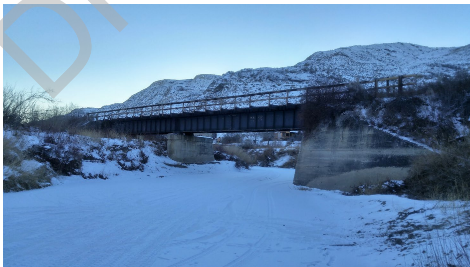
Downstream Side of Bridge
