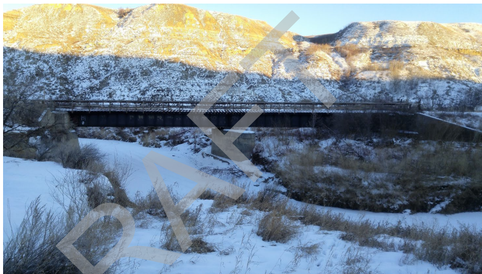
Upstream Side of Bridge
