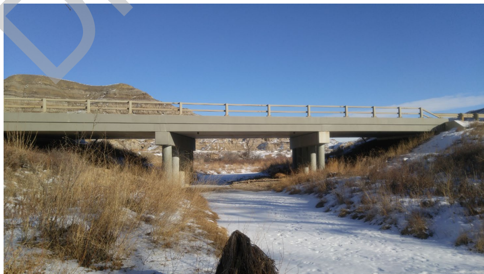
Downstream Side of Bridge
