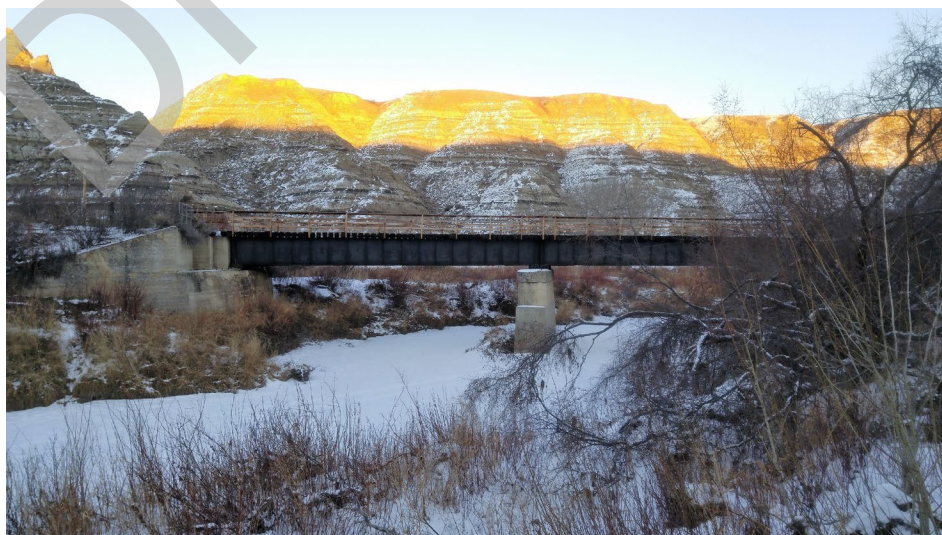
Downstream Side of Bridge
