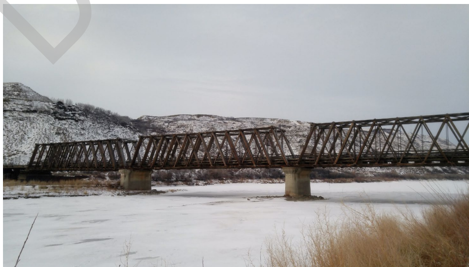
Downstream Side of Bridge
