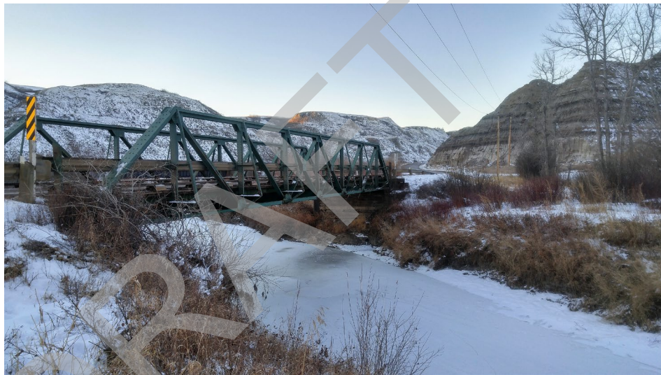
Upstream Side of Bridge
