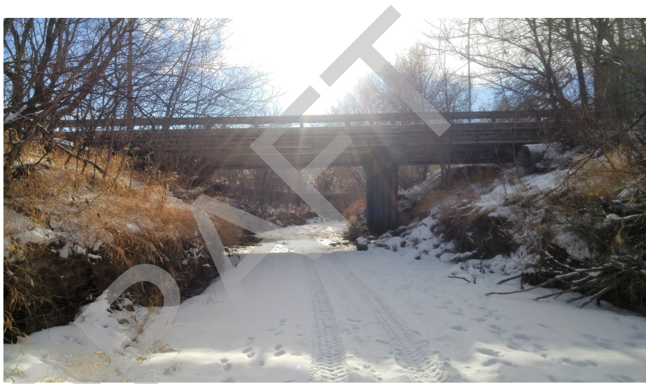
Upstream Side of Bridge
