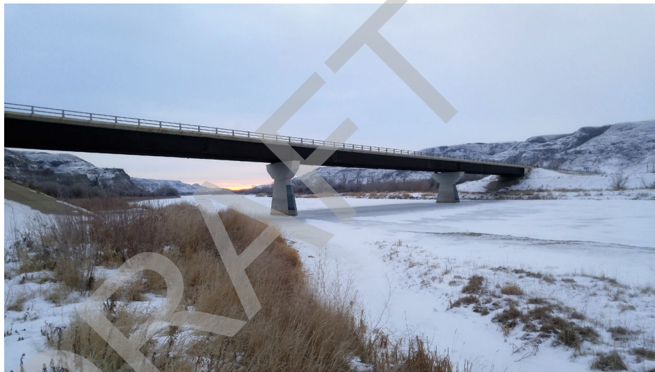
Upstream Side of Bridge
