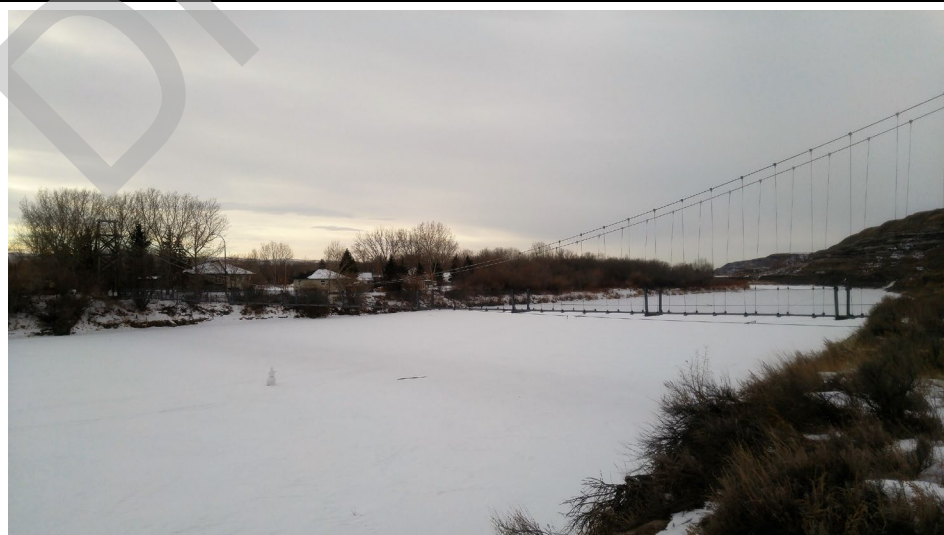
Downstream Side of Bridge
