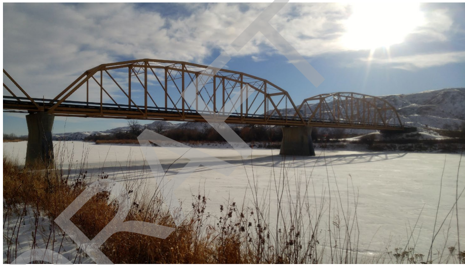
Upstream Side of Bridge
