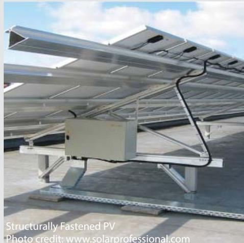
Structurally Fastened PV
