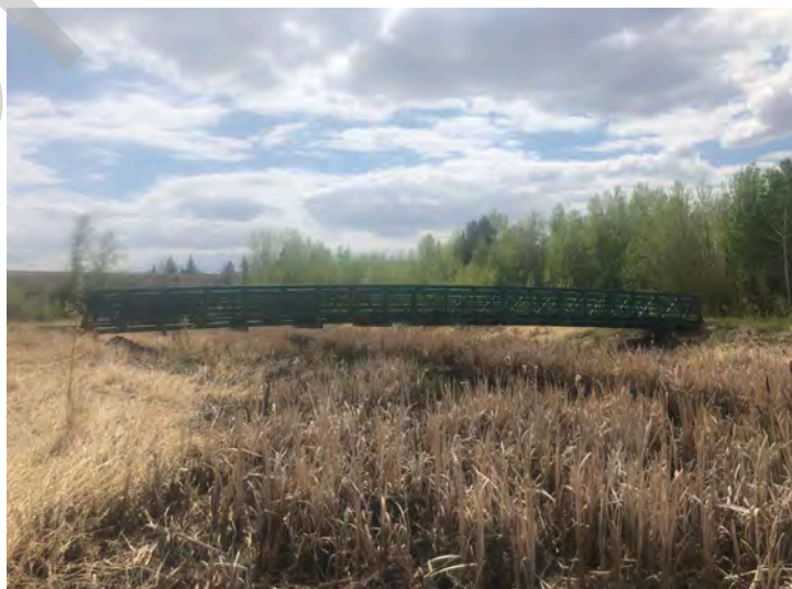
Looking downstream at bridge from left bank
