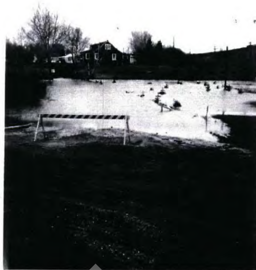
LOOKING WEST, SOUTH OF CPR EMBANKMENT - BRIDGE/ROADWAY FULLY SUBMERGED
