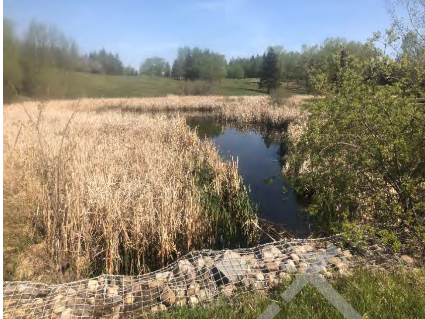
Camrose Creek (upstream view) at 50 th avenue near River Station 12,767 m.
