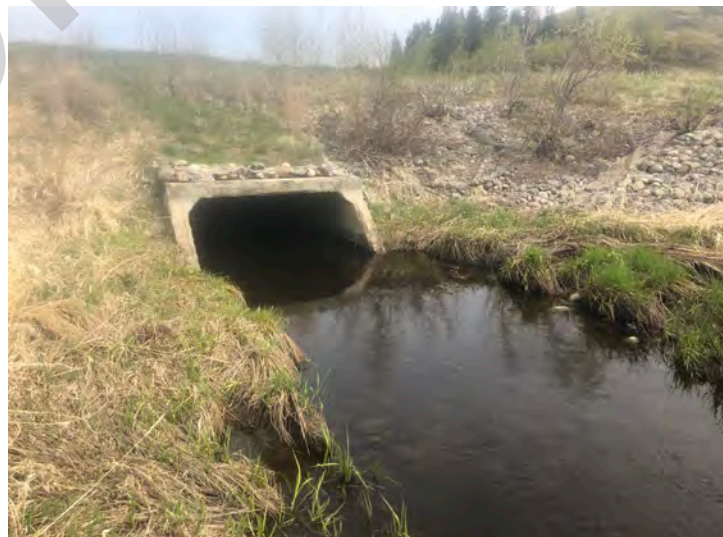
Looking at downstream end of culverts from right bank
