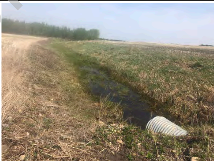
Looking at downstream end of culvert from left bank
