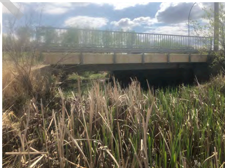
Looking downstream at bridge from left bank
