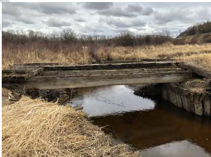
Looking downstream from left bank
