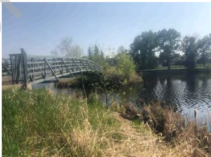
Looking downstream at bridge from left bank
