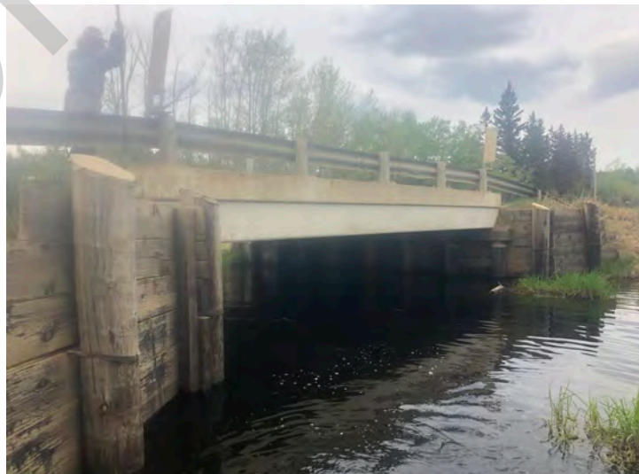
Looking downstream at bridge from left bank
