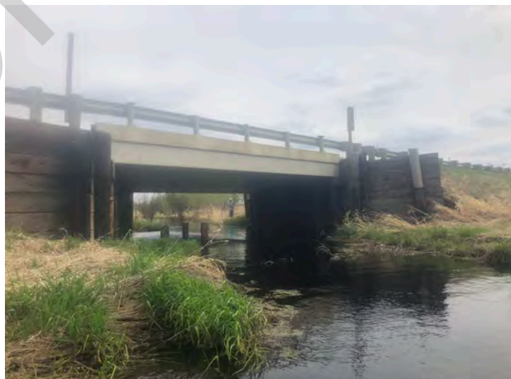
Looking downstream at bridge from right bank
