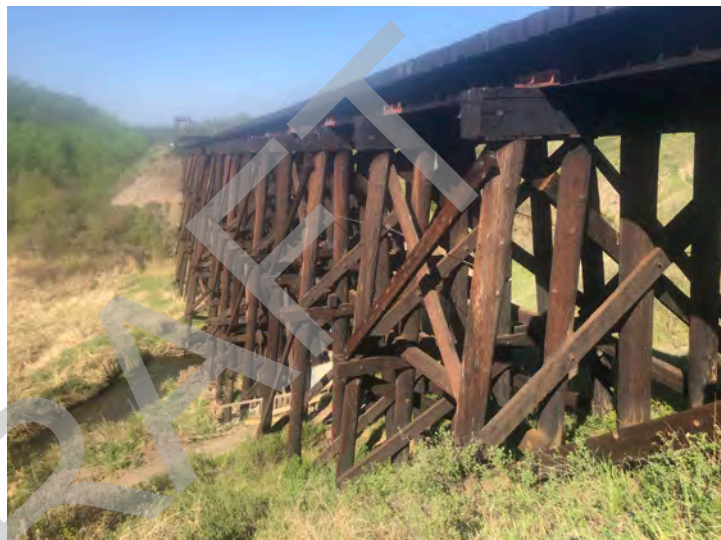
Looking downstream at bridge from right bank
