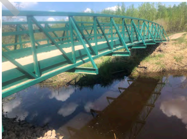
Looking downstream at bridge from left bank
