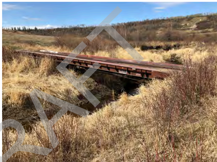
Looking downstream at bridge from right bank
