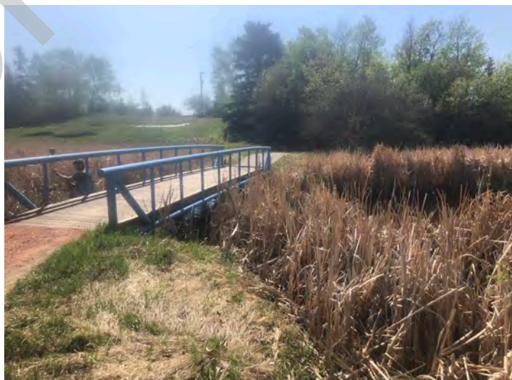
Looking downstream at bridge from left bank
