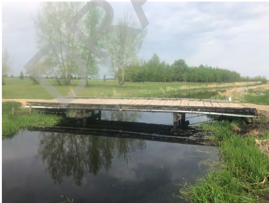
Camrose Creek at a Golf Course Bridge near River Station 17,993 m.
