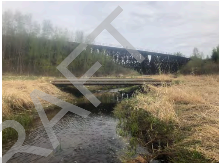
Looking downstream at bridge from center of channel
