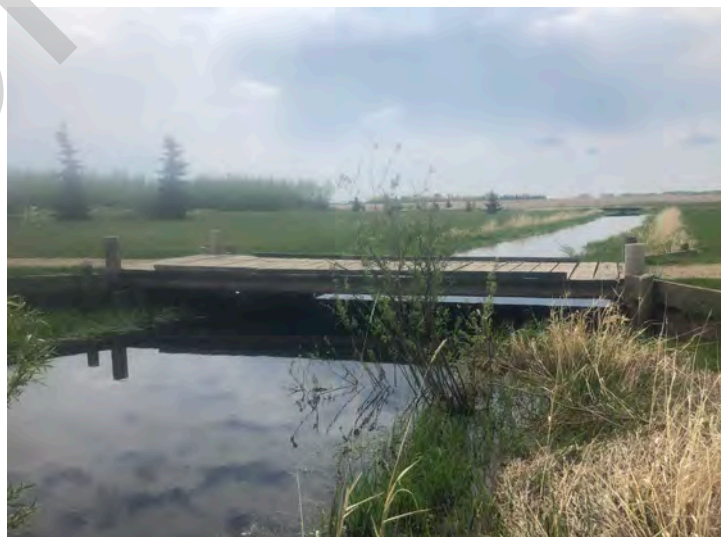
Looking downstream at bridge from right bank
