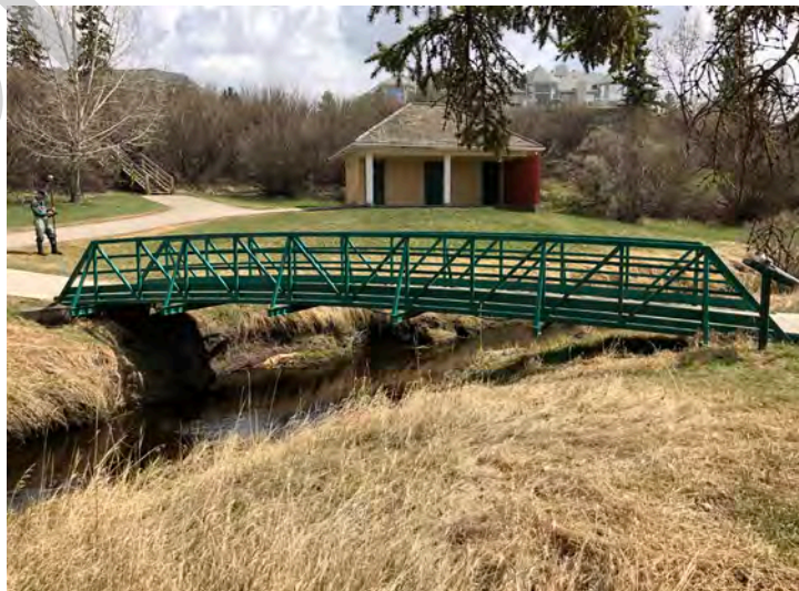
Looking downstream at bridge from right bank
