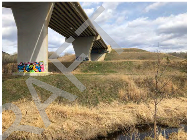
Looking east under bridge from right bank
