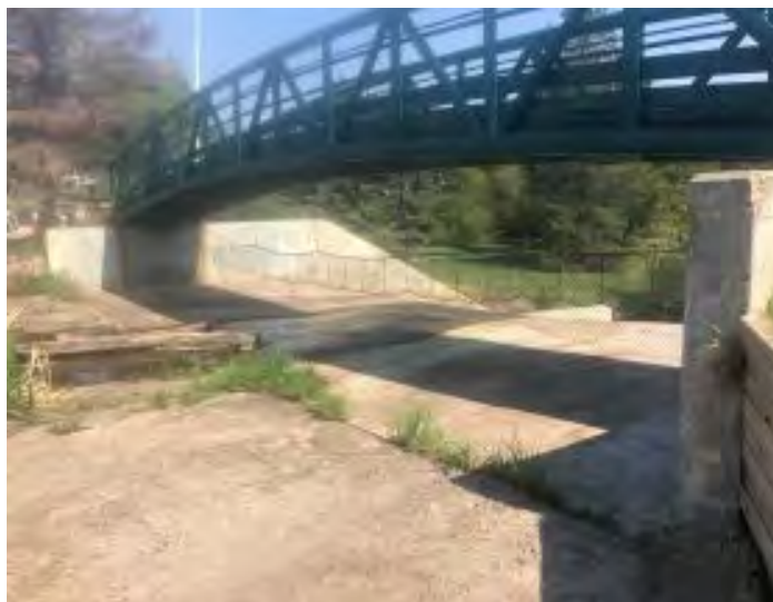
Looking downstream of weir from right bank
