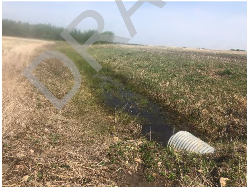
Unnamed Creek (downstream view) near River Station 4,112 m.
