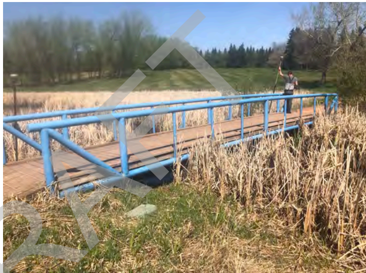
Looking downstream at bridge from left bank
