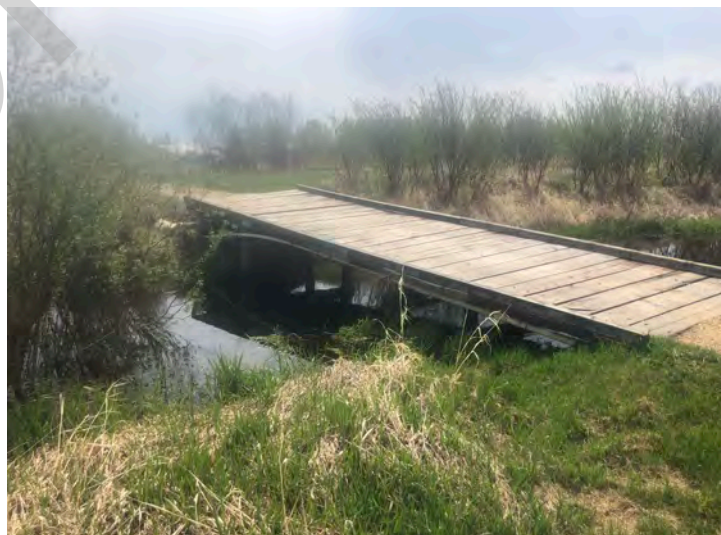
Looking downstream at bridge from right bank
