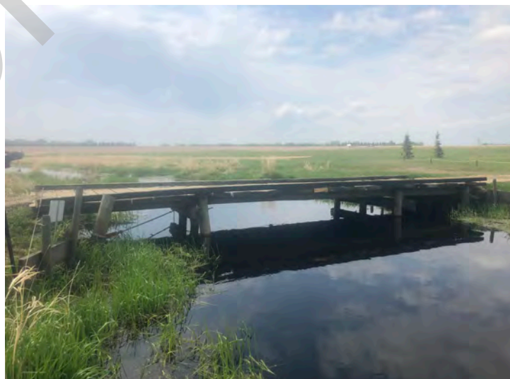
Looking downstream at bridge from left bank
